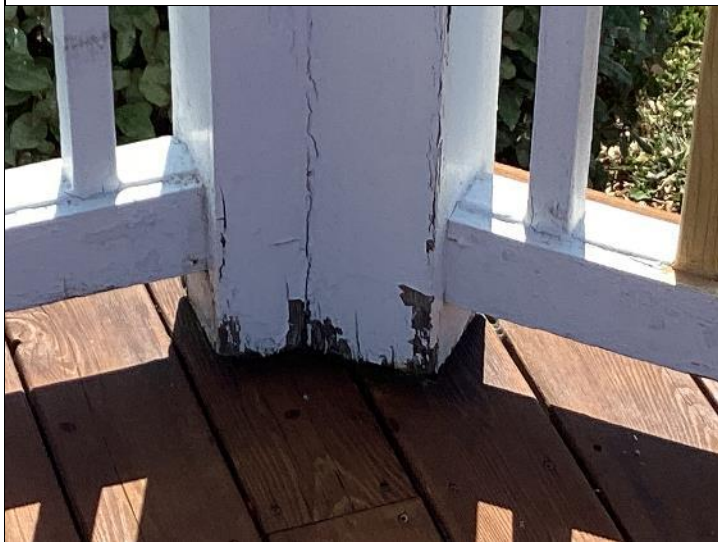
Photo #44: Consideration should be given to properly preparing and painting the wood railings on a cyclical basis to preserve the wood.
