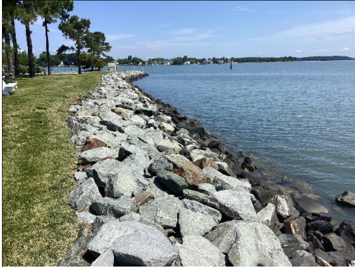
Photo #52: Shoreline riprap. This is likely life of property. A small allowance has been added for maintenance of this seawall.
