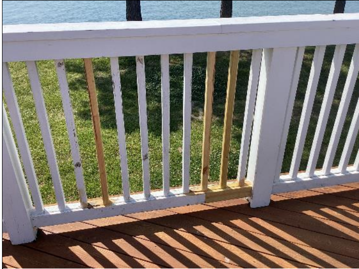
Photo #43: Repairs made to the wood railings.
