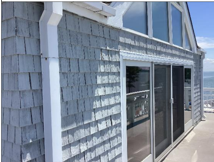
Photo #38: The exterior siding is scheduled for replacement.
