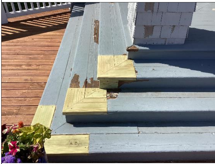
Photo #42: Repairs made to the decking.
