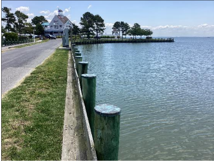
Photo #16: The bulkhead will be replaced sectionally overtime.
