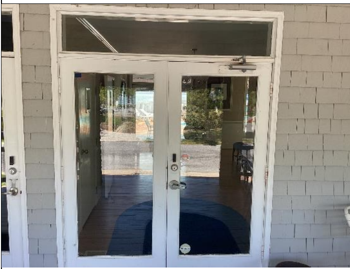
Photo #21: Community building entry.
