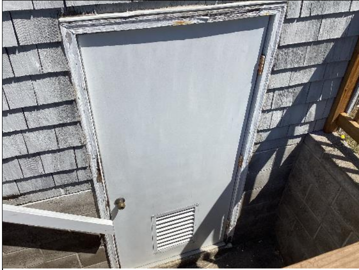
Photo #49: Pool mechanical room door.
