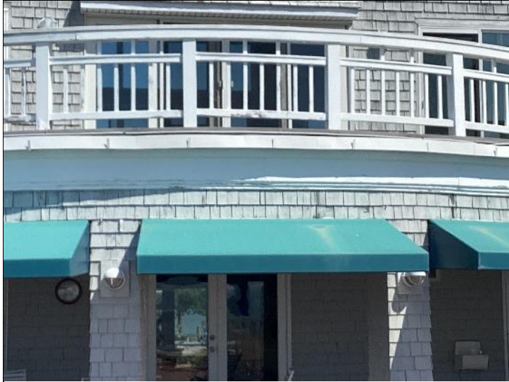
Photo #46: Community buildings awnings.
