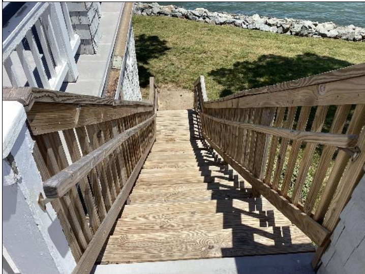
Photo #41: Community building egress stairs.
