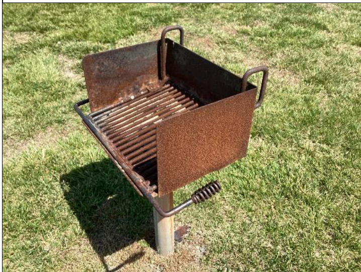
Photo #50: The stationary grills have oxidized. Consideration should be given to painting these on a cyclical basis to preserve the metal.
