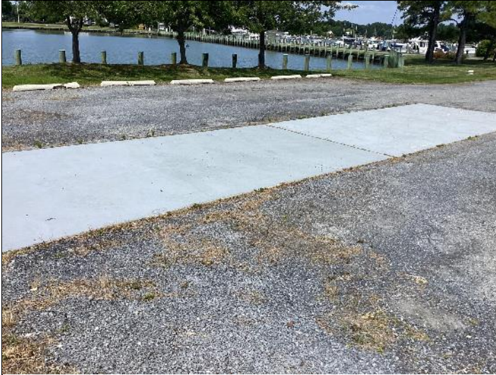
Photo #19: Concrete drive pad.
