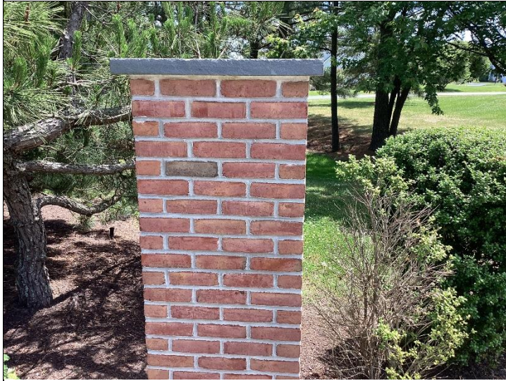
Photo #2: The brick columns were in good condition during our review.
